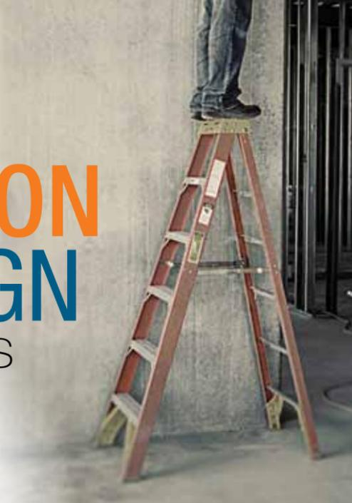
Using ladders on uneven ground, overreaching (below left), working on ladders backwards, missing the bottom step or standing on the top cap (above) are all human-error reasons why ladder accidents are so prevalent in the workplace.
