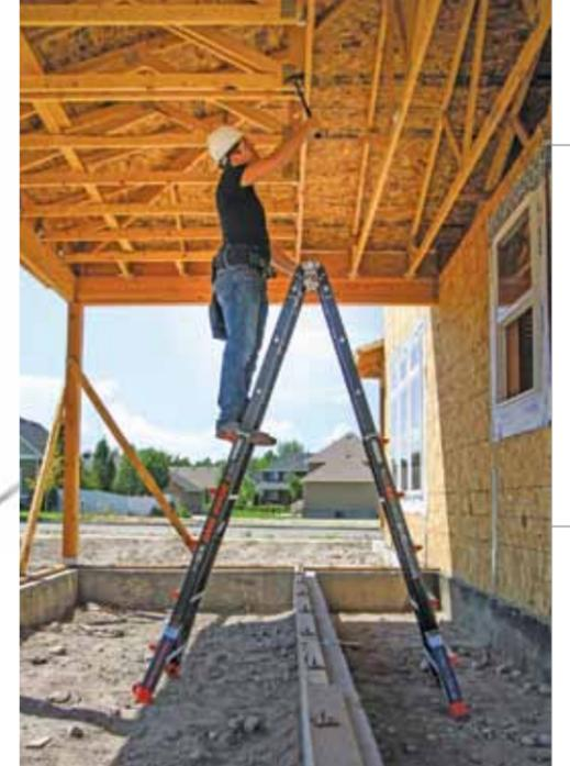
Proper ladder usage can be encouraged by well-engineered ladders that help avoid common accident causes "by design." Adjustable leveling feet, outriggers for stability and cages that enclose workers all help minimize user-error risks of accident.
