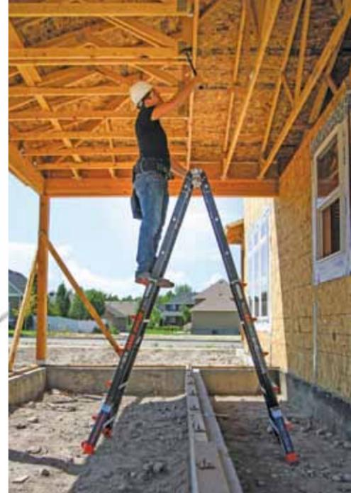
Proper ladder usage can be encouraged by well-engineered ladders that help avoid common accident causes "by design." Adjustable leveling feet, outriggers for stability and cages that enclose workers all help minimize user-error risks of accident.
