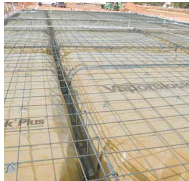
Strong Man VaporBlock Plus 20 is a seven-layer barrier made from state-of-the-art polyethylene and barrier resins. It provides unmatched impact strength and superior resistance to gas and moisture transmission.
