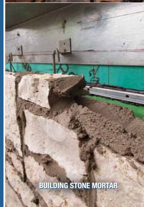
SETTING BED MORTAR-DRY PACK
