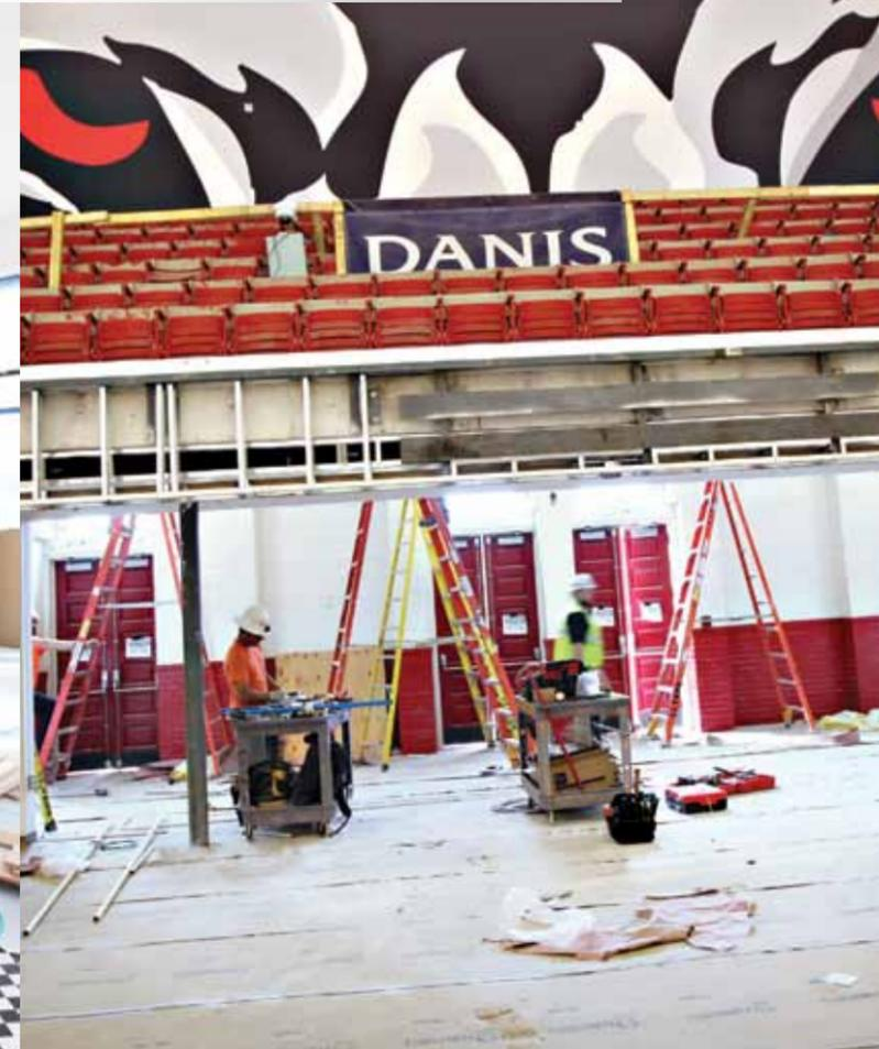
Trimaco’s FloorShell is a heavy duty construction board that is liquid resistant and breathable to allow surfaces to continue curing. Plus, the scored edge makes it simple to fold and protect baseboards and walls. Strong enough for forklifts!
