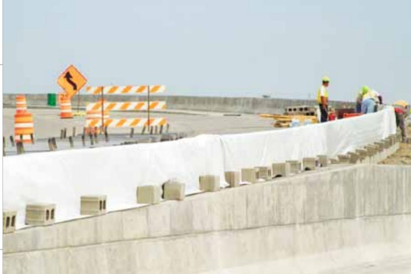
**Conkure Wet Curing Blanket** from Strong-man consists of a highly absorbent synthetic needle-punched fabric coated with a white reflective film. Unlike burlap, it will not rot or mildew.
