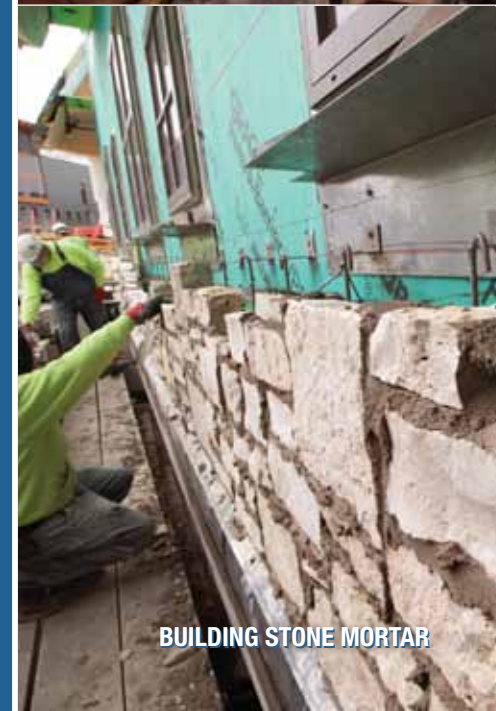
SETTING BED MORTAR-DRY PACK
