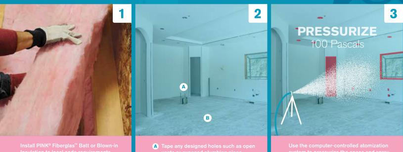
Insulation to local code requirements. Complete drywall installation and first mud application.\*
