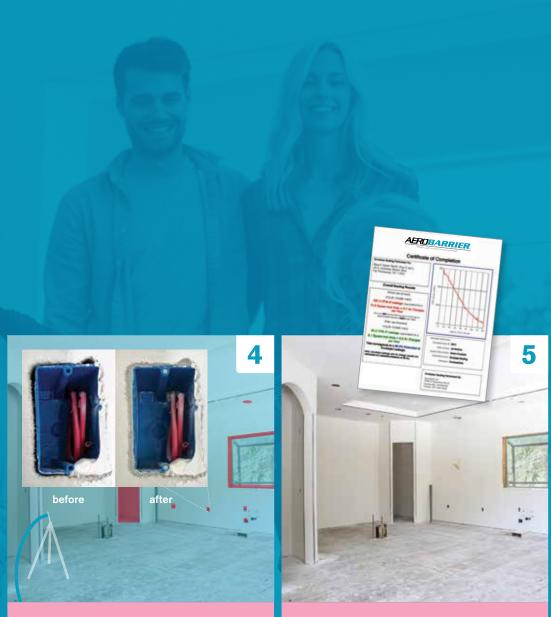
Allow the particles to build up around any gaps and holes to seal leakage areas without coating surfaces.
